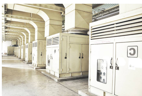
Natural gas compressors
