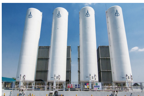
Natural gas quality improvement station
