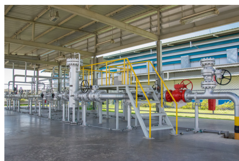
Metering system at the natural gas quality improvement station
