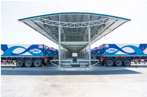
Natural gas refill station for transportation
